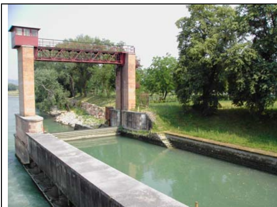
Picture 3: The unused lock at Chievo dam. The gantry hoist and sliding gate are located at the downstream end .
