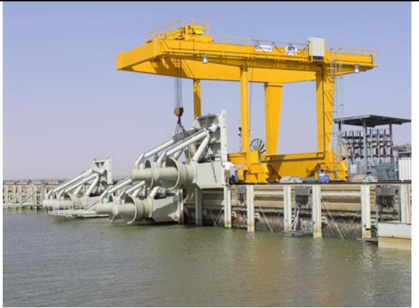
Picture2: Photo of the modules in raised condition
