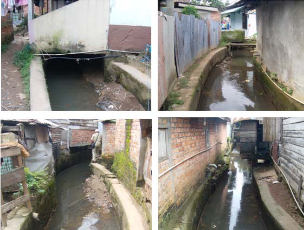
Figure 14. Photo's of drainage channel conditions at the upstream of retention basin
