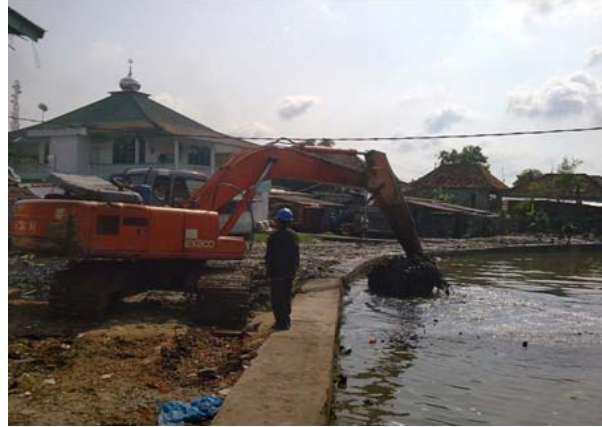
Figure 12. Normalization activity of the drainage system
