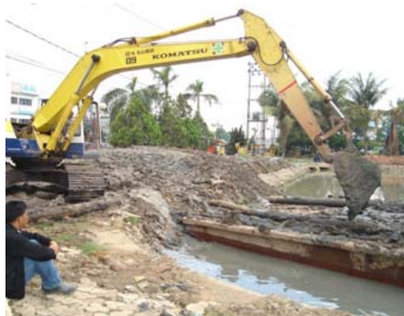
Figure 14. Dredging activity at Siti Khodijah retention basin
