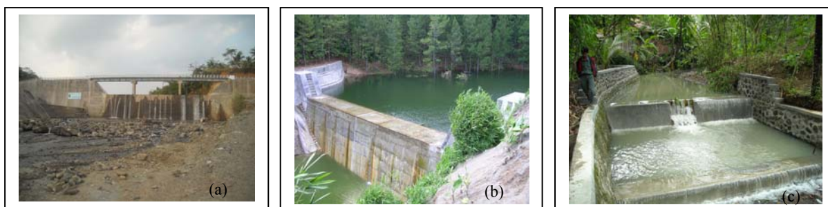
Fig. 11. Examples of constructing large, medium and small size of sedimentation control built at some tributaries in the upper watershed of the dams
