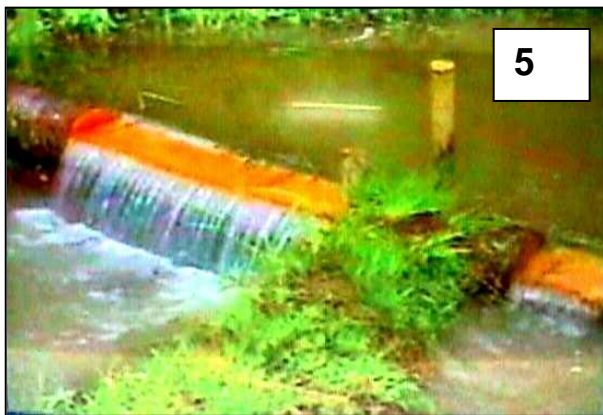
Figure 5. Simple water measurement device ( tektek ) invented by Subak in Bali.
