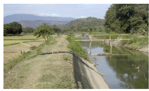
Fig. 8 Photos of water illegal abstraction by using plastic hose on main canal Tabo-Tabo
