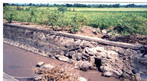
Fig. 9 Photo of water illegal abstraction from secondary canal Bulo-Bulo, Kelara Karalloe I/A
