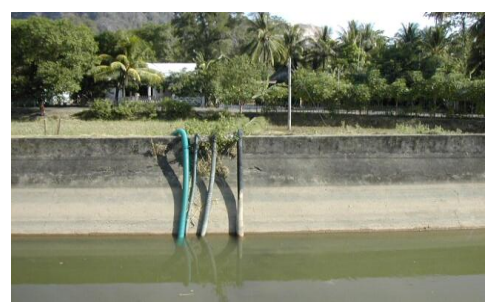
Fig. 8 Photos of water illegal abstraction by using plastic hose on main canal Tabo-Tabo
