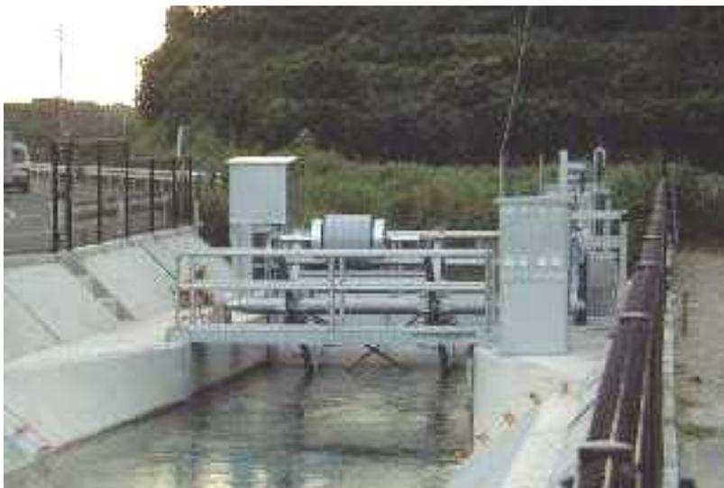
Fig.4 Mechanical Automatic Check-Gate
