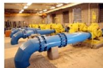
Pumping station site
