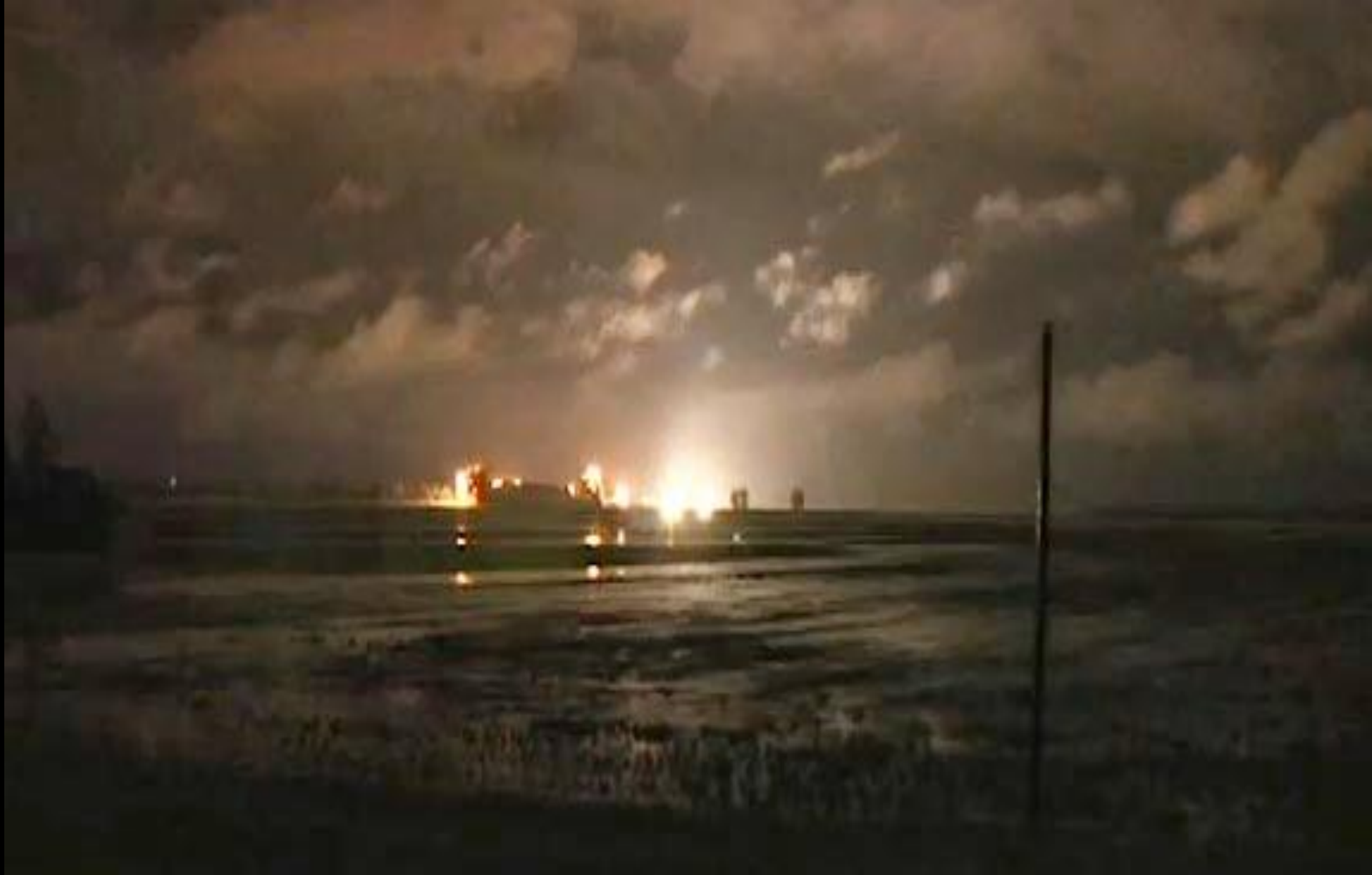
Army Corps of Engineers 's demolition of the Birds Point levee on the Mississippi River on May 2, 2011.
