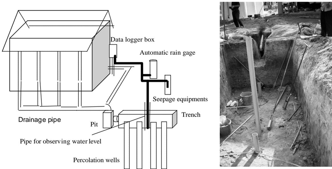
**Fig. 24** Outline of equipment in the field **Picture 1** Recharge system (before gravel filling)
